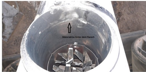
Failure on part
