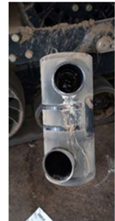
Removed failed part
