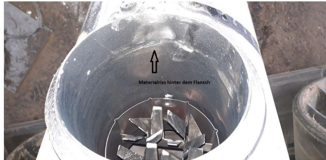
Failure on part
